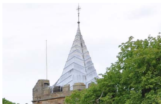
FOUND MATERIALS: new zinc roof with seams to match St Deiniol's church's lead spire
